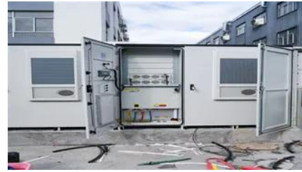
Nur Bukhara Solar and Battery Project: Uzbekistan's First Utility-Scale
