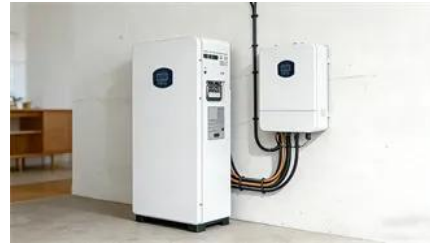
Solar container communication station lead-acid battery parameters
