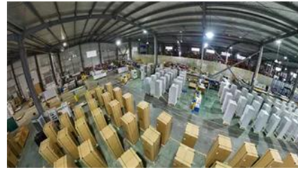
World's largest PV-CSP plant under construction in China
