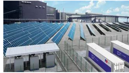
Flywheel Energy Storage: Grid Frequency Regulation Economics
