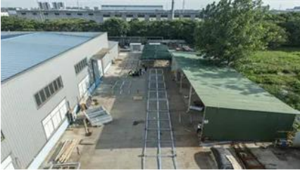
Outdoor Energy Storage System Cabinets , EPC Energy
