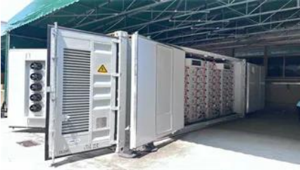
Namibia photovoltaic power station energy storage battery
