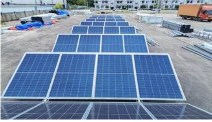
Photovoltaic Energy Storage Cabinet Manufacturer in Salzburg.
